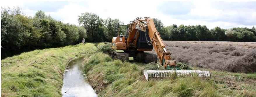
Picture 4.4: Servicing of highly effective flood defence in 2011
